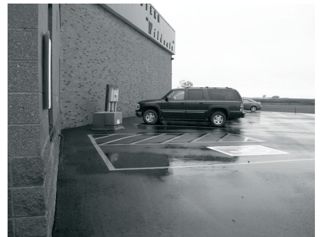
This summer the high school parking lot was paved.
